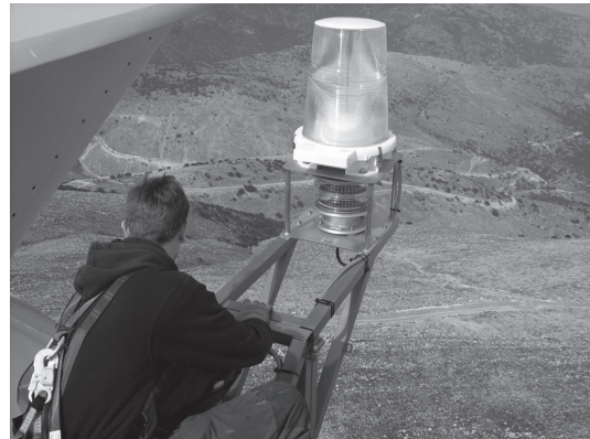
Figure 1. The W/T service technician at work.
